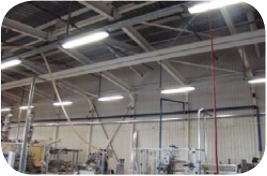
Industrial and stores areas, housing and utilities
